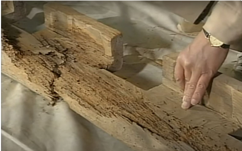
Traditional conservation techniques for wood
